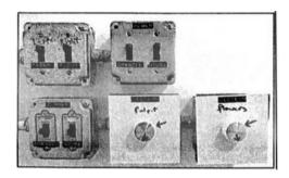
Spotlight switches (rheostats) are located in the Pulpit side hallway. To turn OFF, rotate dials counterclockwise until you feel a click. When turned OFF, the arrow on the dial will be pointing to 6 o'clock.
